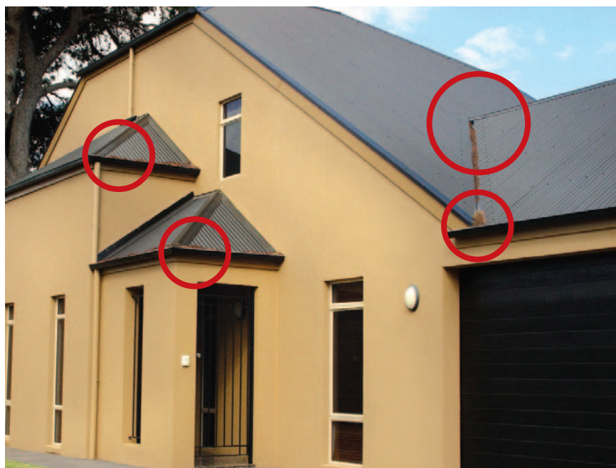
Above: Combustible debris can accumulate in roof valleys and gutters.
