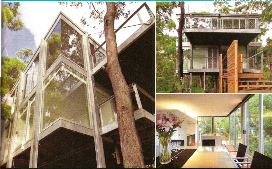
EXTERNALS: galvanised steel frame, clear anodised window frames glazed with Pilkington Activ self-cleaning glass, concrete slab floor, Colorbond roofing INTERNALS: steel and timber frame lined with plasterboard
